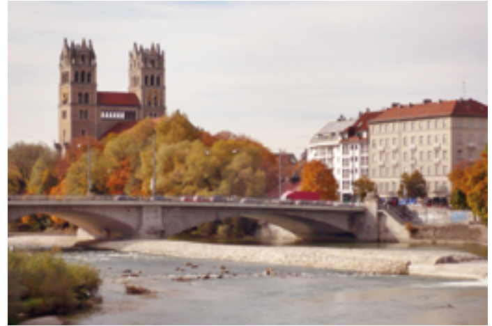
Reichenbach bridge and Church of St. Maximilian
